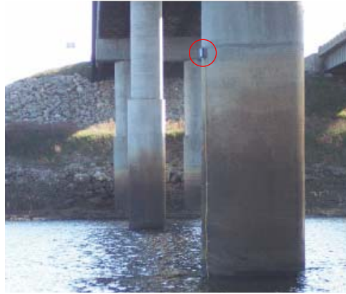
Fig. 3. Installation on Bridge A6531 in Osage Beach, MO.
