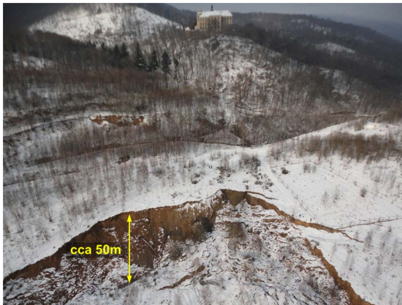
Fig. 7 Landslides at the pillar protecting the castle [11]
