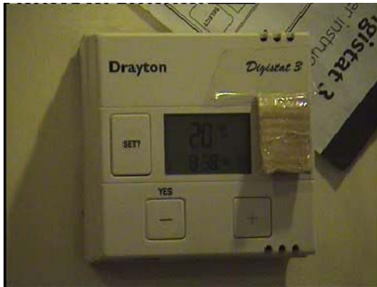
Fig. 1. Heating control modified using principles from aircraft cockpit design
