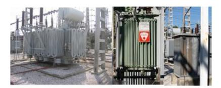
Fig. 2. Protected substation components: HV/MV Power Transformer (left), Neutral Reactance (centre) and Neutral Resistor (right).
